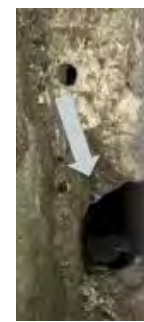
Fig. 3 (above) Pilot hole to 1x1m typically takes ~8 minutes.
