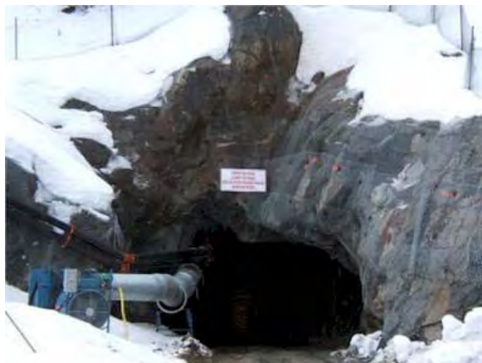
Fig. 15 (above) Rocmec 1 portal
