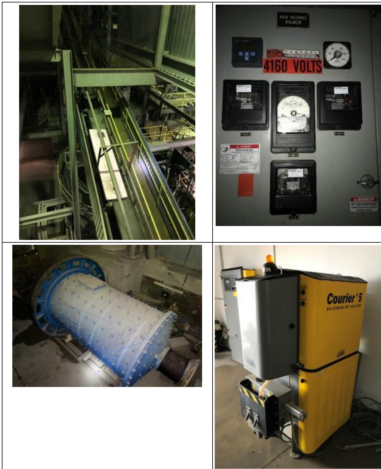
Figure 18-21: Selected Warehouse Assets
