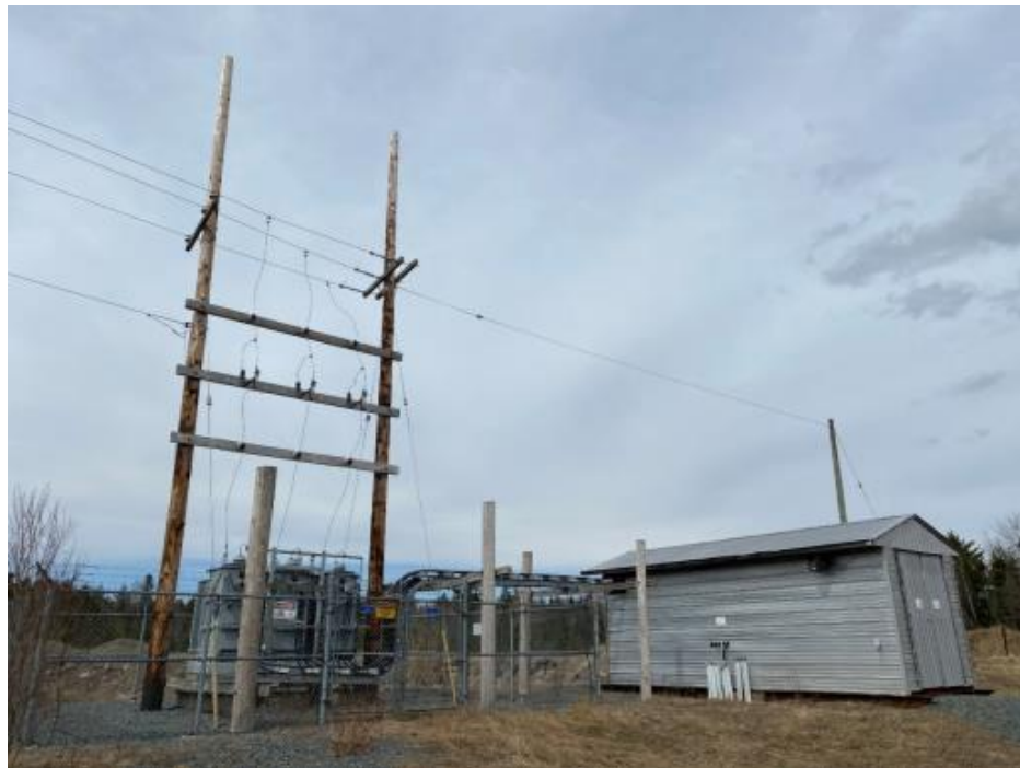
Figure 18-5: Mine dewatering transformer and substation
