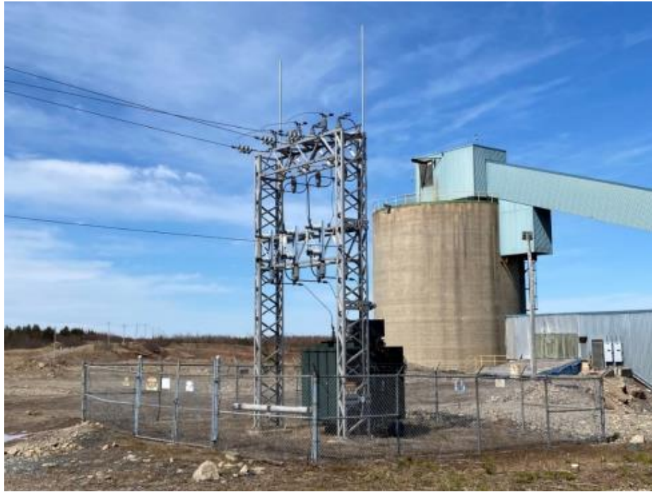
Figure 18-5: Mine dewatering transformer and substation
