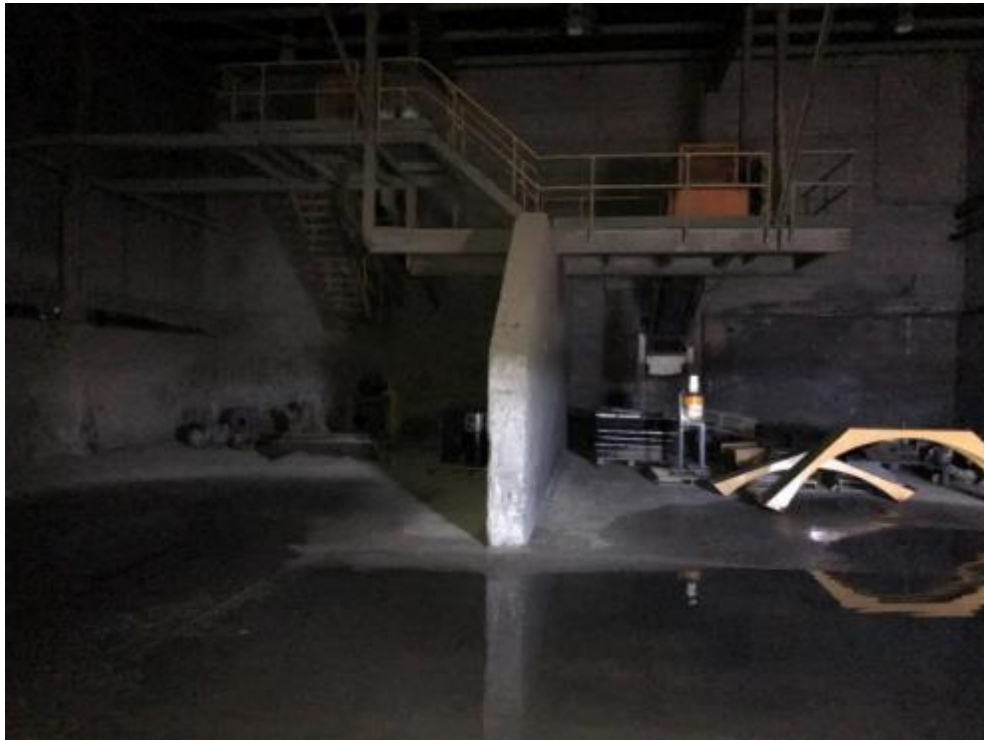
Figure 18-40: Concentrate Loadout Area
