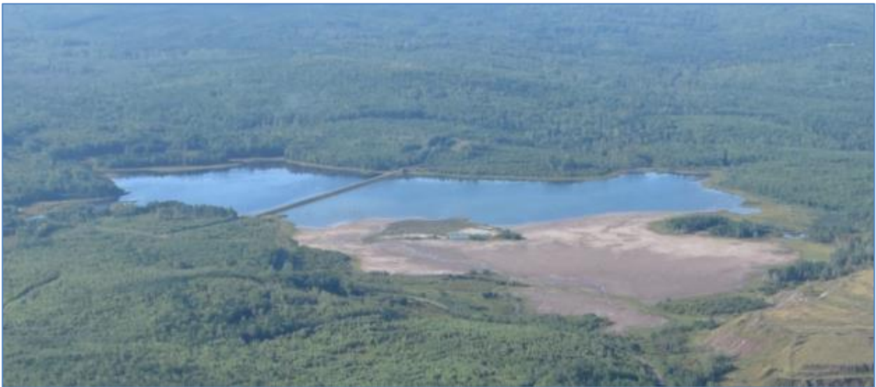
Figure 18-47: Tailings Storage Facility
