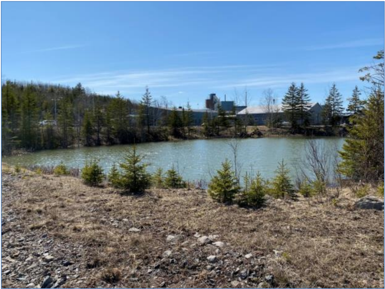
Figure 18-12: Storm Water Pond
