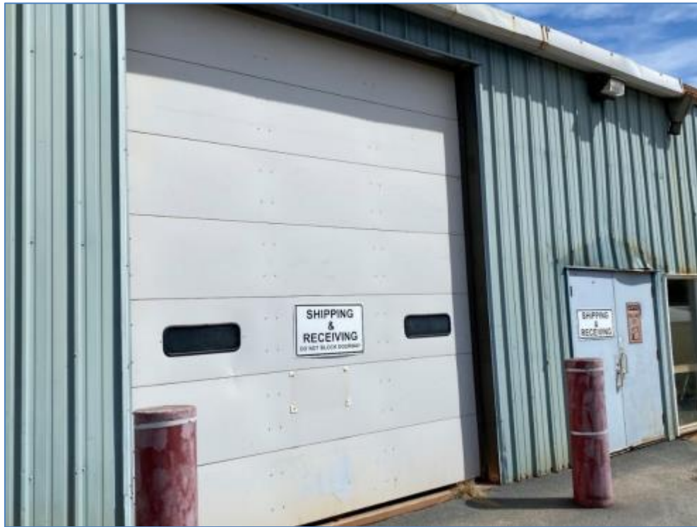
Figure 18-17: Site Warehouse Receiving Bay
