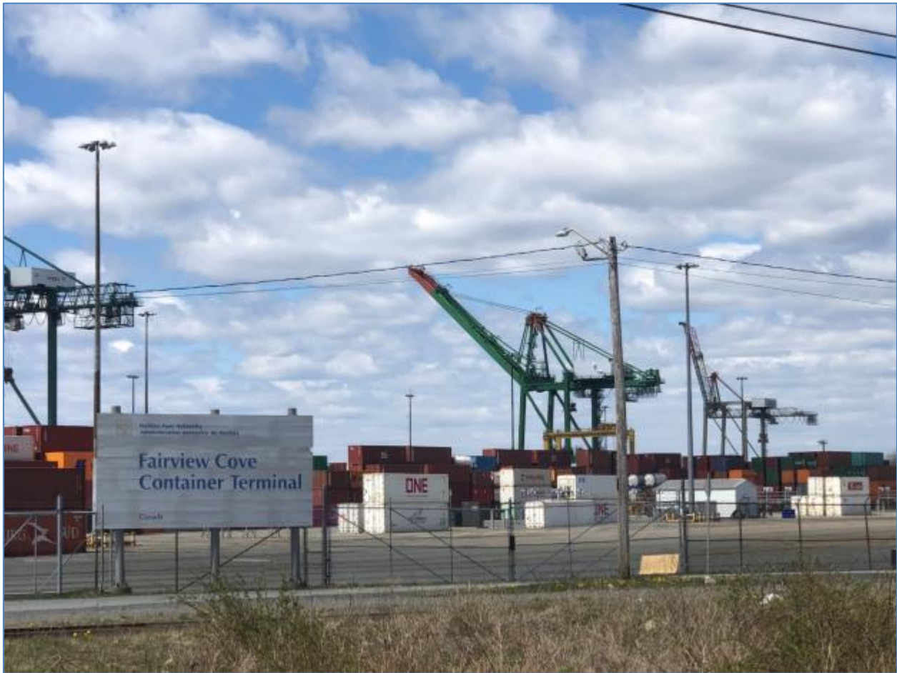
Figure 18-75: Fairview Cove Container Terminal
