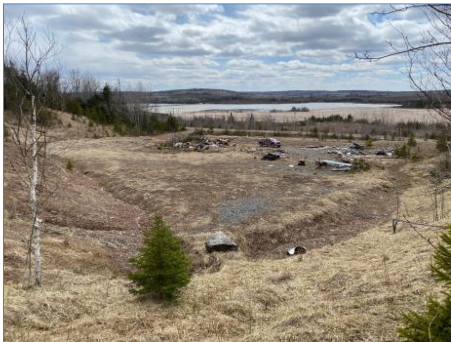
Figure 18-63: Secondary Laydown Area (Proposed New Reservoir location)
