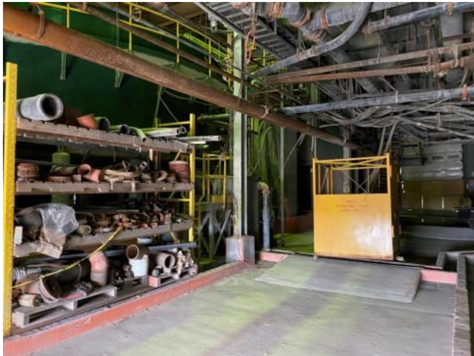
Figure 18-46: Large Ground Floor Maintenance Bays
