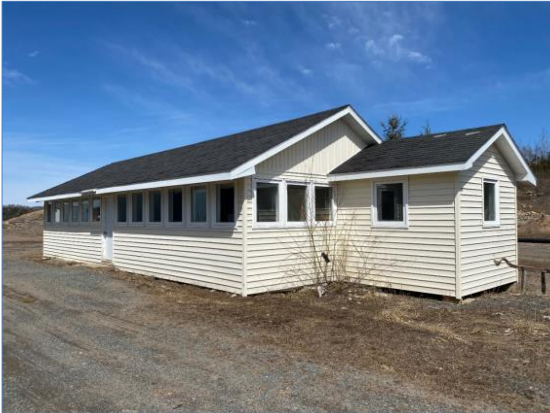
Figure 18-27: Core Preparation Building
