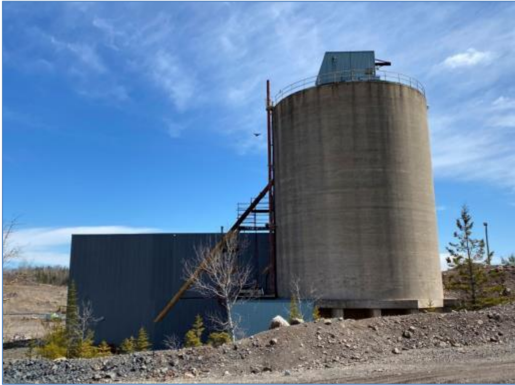
Figure 18-33: Existing Mill Fine-Ore-Bin (Silo)
