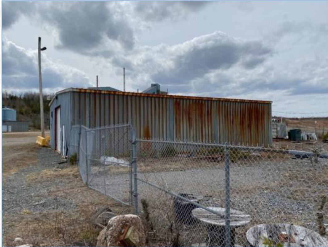
Figure 18-51: Cold Warehouse and Storage Yard
