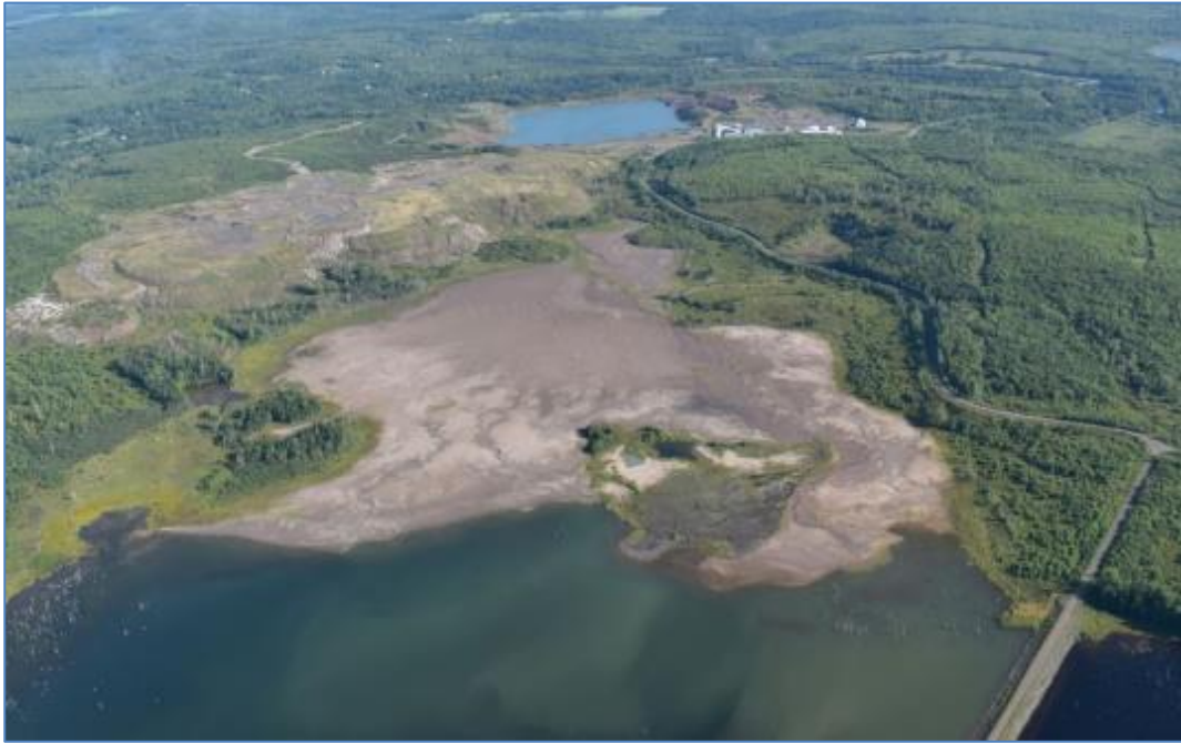
Figure 18-56: Tailings Storage Pond
