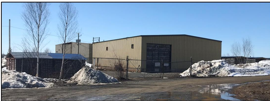
Figure 12.3 - View of the old mill facility along with some of the well-maintained outside storage racks
