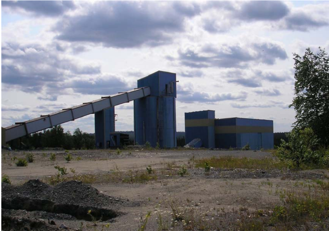
Figure 15.1: Former Chimo Gold Mine (July 2006).
