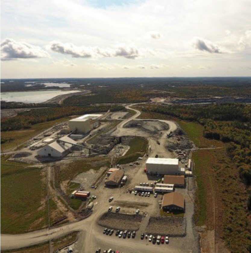
Figure 18 Areal view of the Moose River open pit mine.
