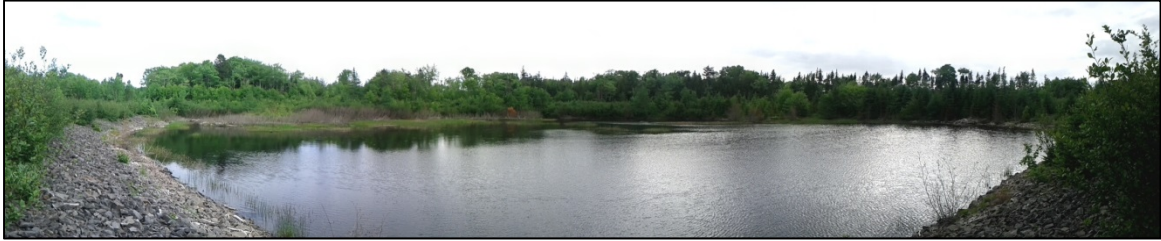
Figure 5-3 - Mooseland Settling Pond, Looking Southwest
