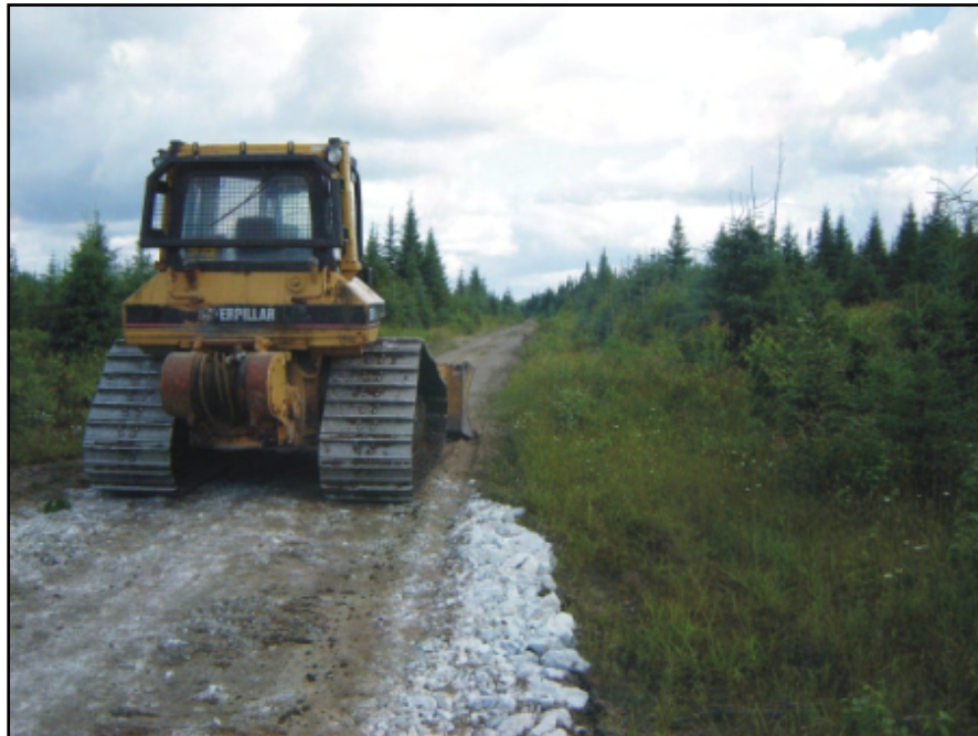
Figure 5.1 View of Access Road and General Physiography, Looking North
